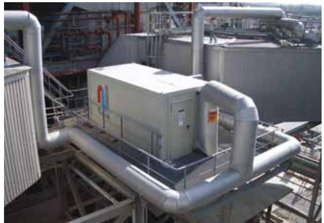
**FGC unit installed between the flue gas ducts on a 575 MW boiler. Typical dosage rate: 15 kg/h. The result: Solid emission <math>< 12 \text{ mg/Nm}\_3</math>**
