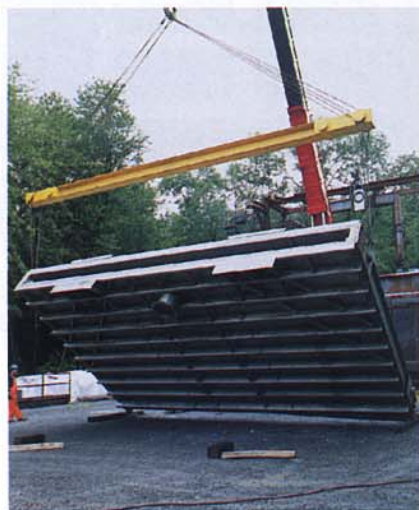
The bonnet serves as an extension to the ductwork, assuring zero leakage to atmosphere under all conditions.
