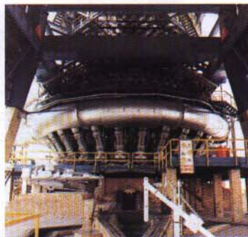
Teyere stock expansion joints for a blast furnace. Iron and steel industry applications also include hot and cold blast mains, gas mains and fume extraction systems.
