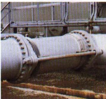
Double tied bellows for petroleum tank settlement. The bellows accommodate tank settlement and other vertical or lateral movements, minimizing stress on both the tank walls and adjoining pipework.
